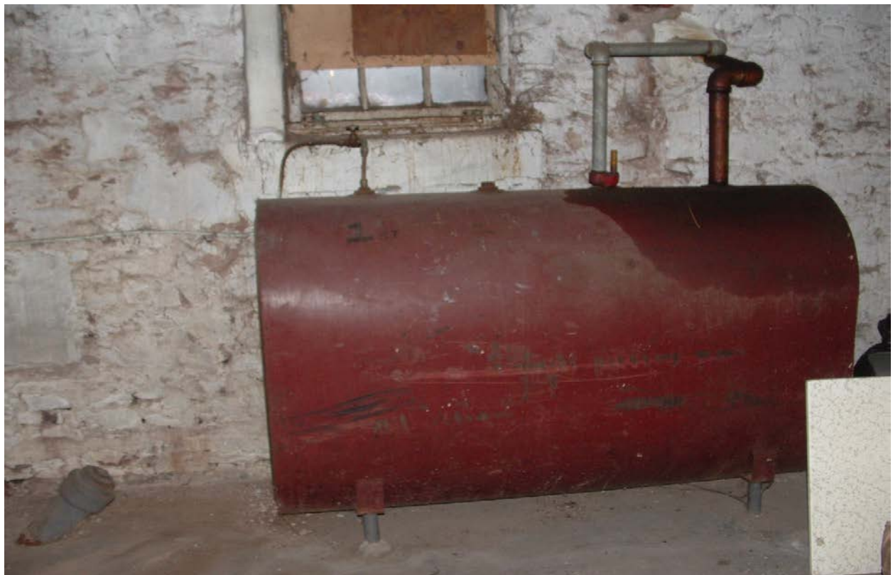
Photo 2 AOC-1 - 275-gallon heating oil AST at 15 Fourth Street
