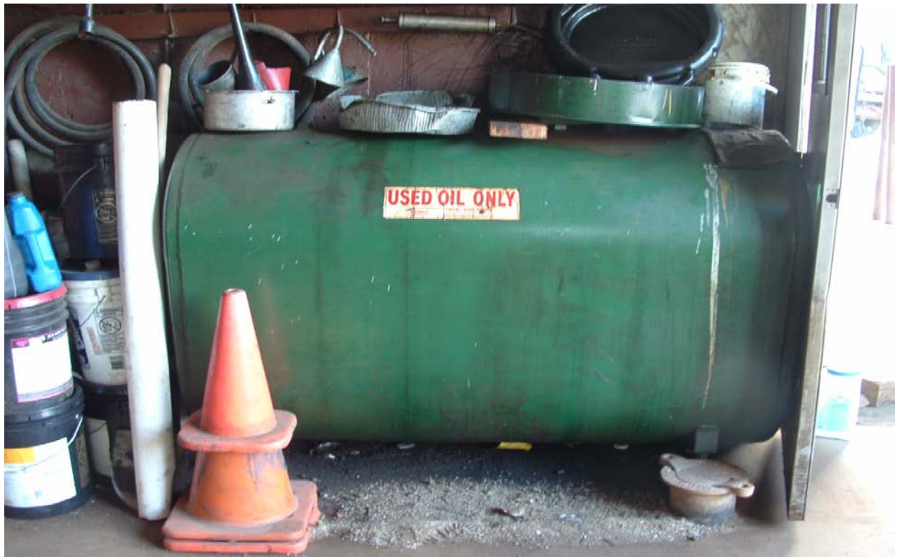
Photo 1 AOC-1 - 275-gallon used oil AST at 13 Fourth Street
