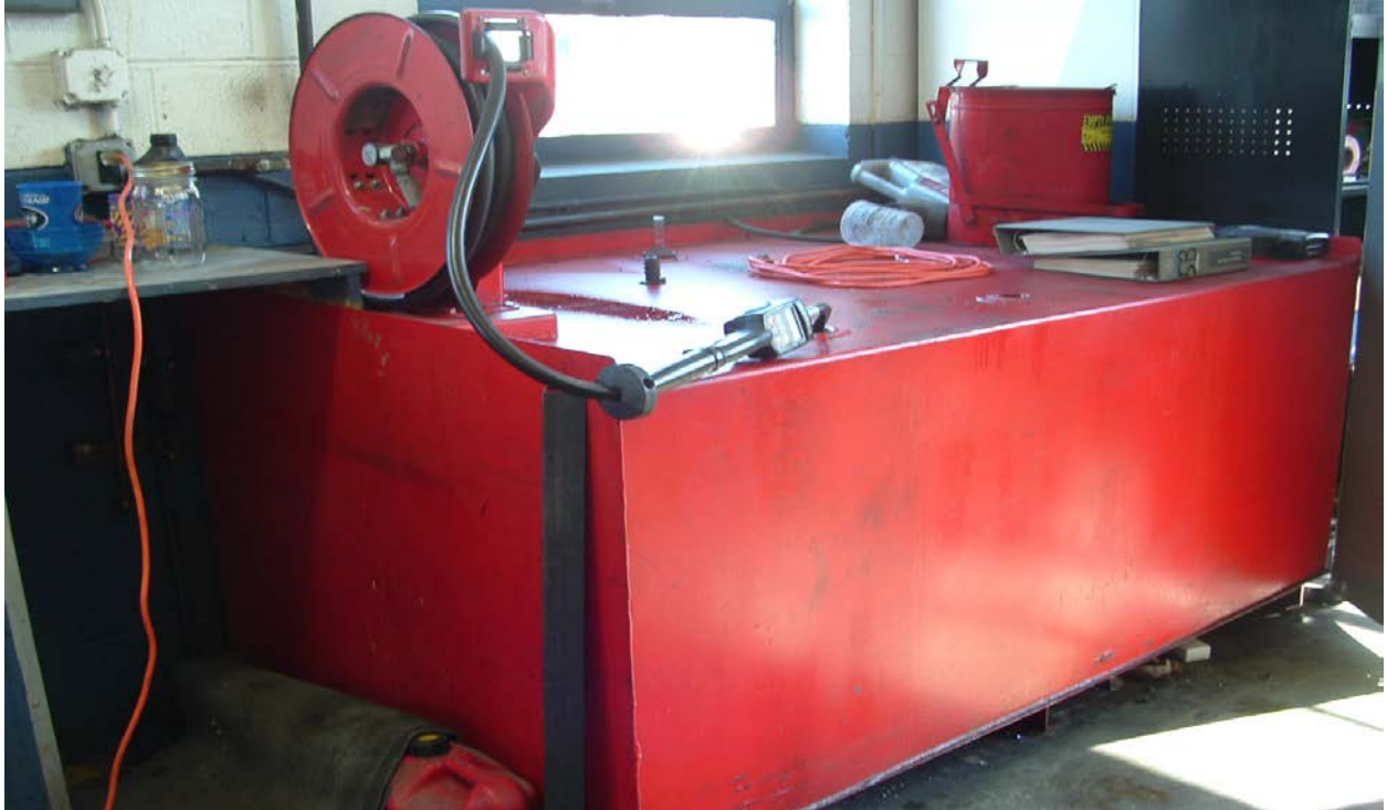
Photo 5 AOC-1 - 500+gallon motor oil AST at 209 Valley Street
