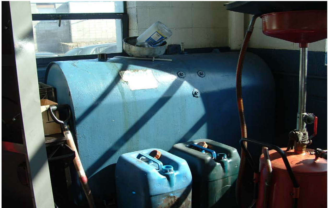
Photo 4 AOC-1 - 275-gallon used oil AST at 209 Valley Street
