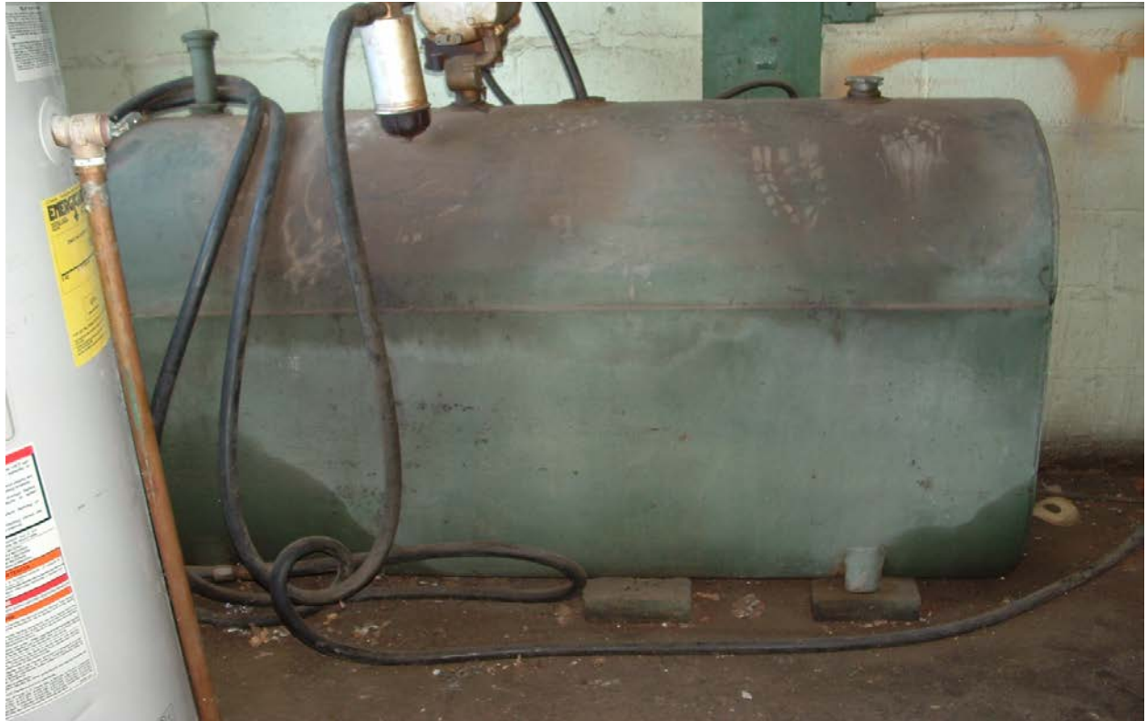
Photo 3 AOC-1 - 275-gallon diesel fuel AST at 16 Fourth Street
