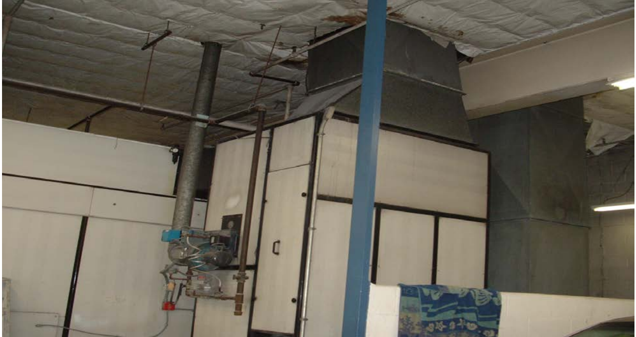
Photo 12 AOC-6 - Spray Booth exhaust system at 209 Valley Street
