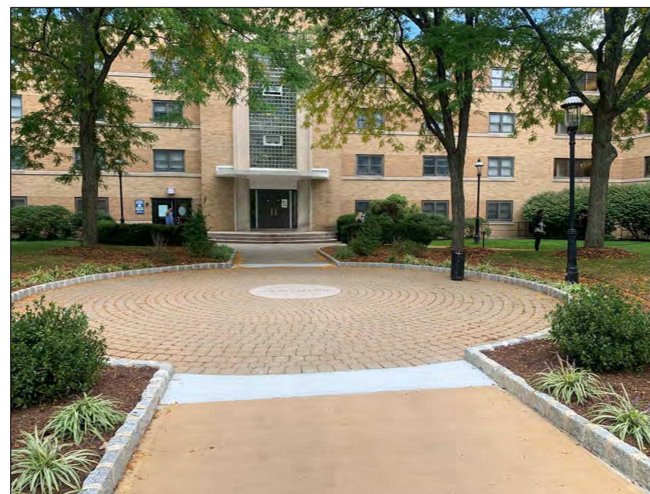
EXISTING BOLAND HALL BUILDING ENTRANCE
